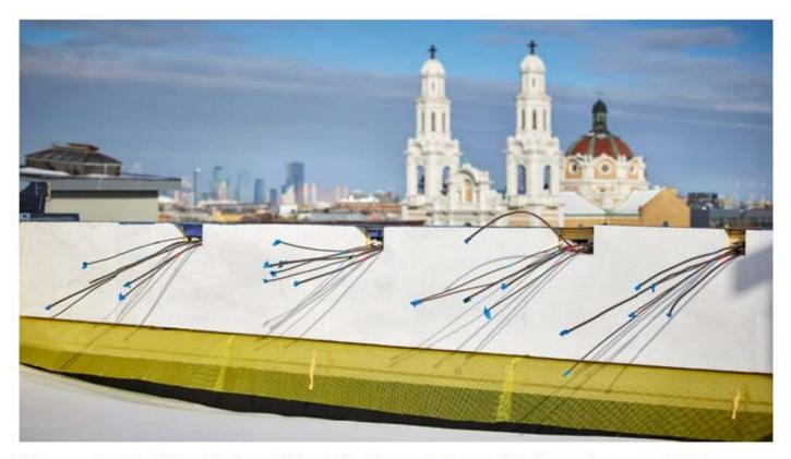
The apartments of Casa Pasiva will have heating and air-conditioning units connected to a system of ducts and refrigerant lines that snake up the walls and connect to a rooftop ventilator. John Muggenborg for The New York Times
